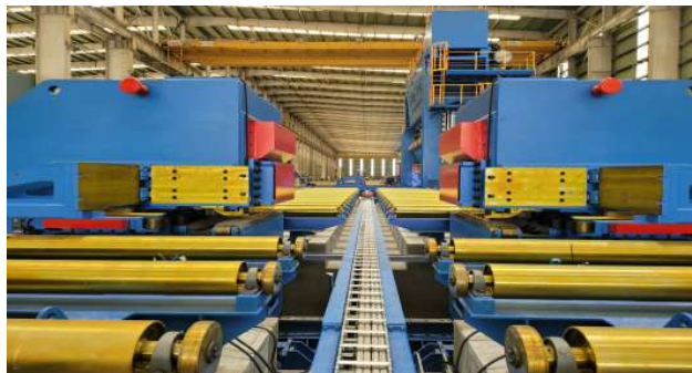
On-site Installation of Pre-bending Machine
