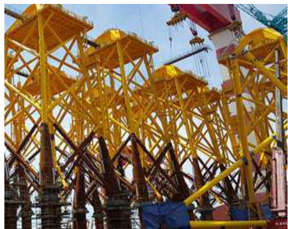
Jacket fabrication completed (Storage yard for jacket products)
